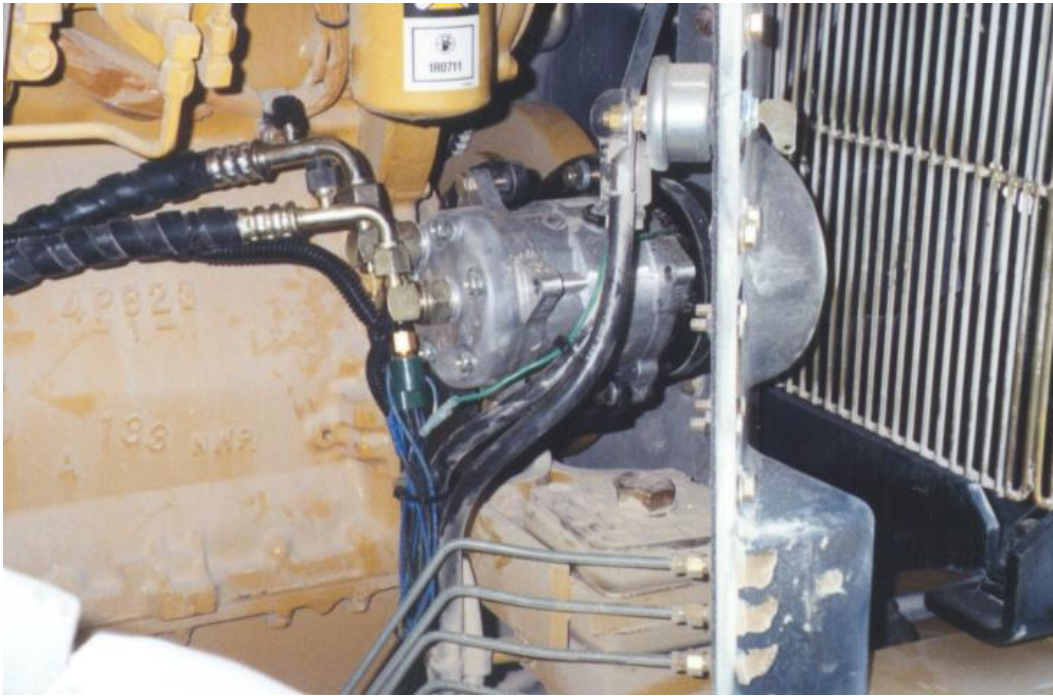
Compressor mount in place.
